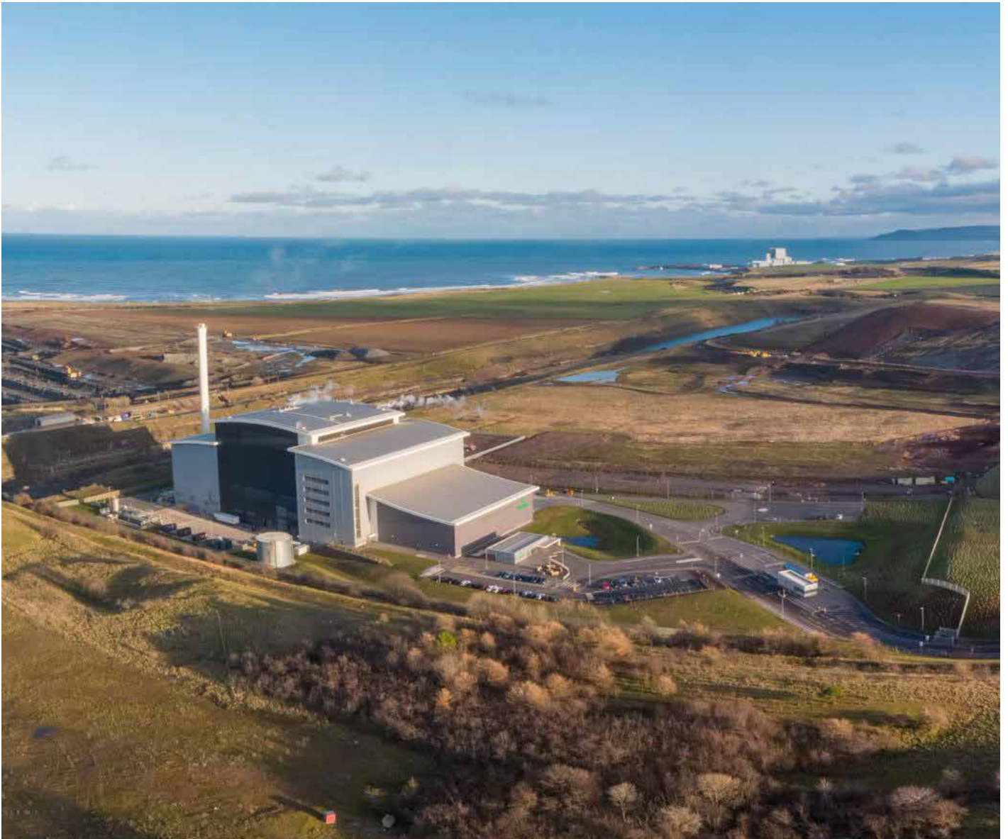
View of the whole site and landfill
